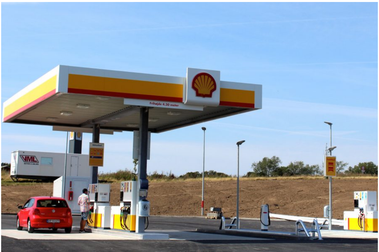
Den nye Shell tank i Business Park Vordingborg
